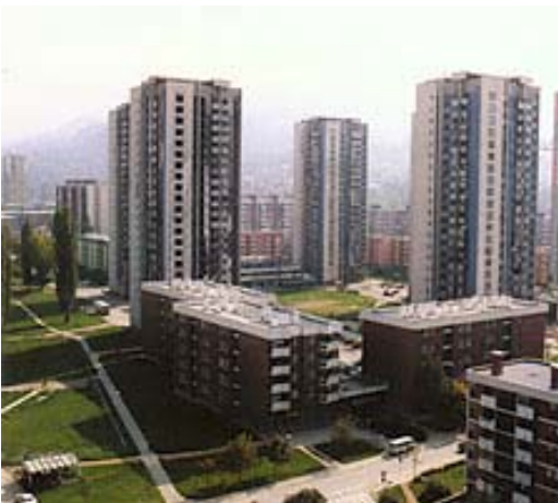
Creating sense of normality: Cleaning the rubble and fixing facades of buildings in Sarajevo
